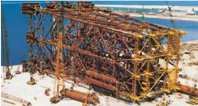
Offshore plant construction: platform
